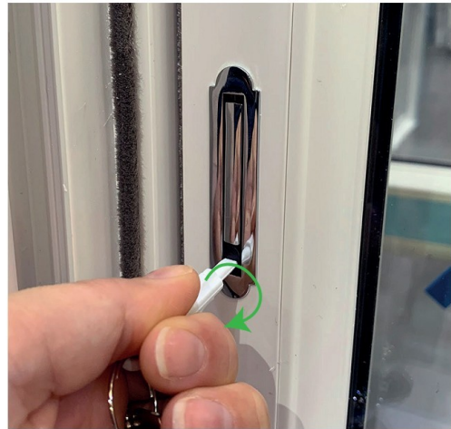
Fit key into cam and turn clockwise to open restrictor
