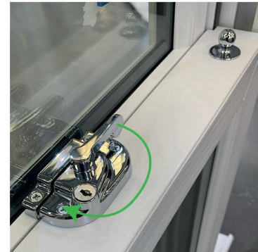
Rotate arm to lock window (CLOSED POSITION) Insert keys and lock (if required)
